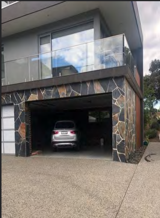
Garage / property overview
